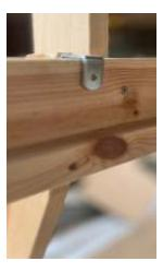
Using the two ladder hooks now attach to the top of each ladder strut, attaching to the slanted inside cut edge, See PIC1 Locate the hooks and attach using the small screw(L). Now hook the ladder over the side rail, this is designed to be tight to prevent movement. You may need to gently tap with a mallet..
