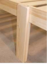
The centre leg will hover slightly off the floor, when the bed is in use it will move down and support the bed. This is to protect the leg if the bed moves.
