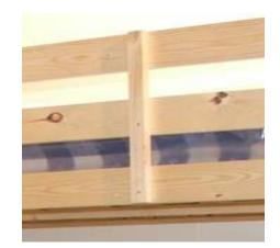
These two rails prevent the guard rails from being forced apart, very important. Using a tape measure find the centre of the back guard rail and centre of the front guard rail. Make a small pencil mark. Then attach each guard rail support to the front using the base slat screw (E) provided. These cover both the two guard rails and secure onto the side rail.
