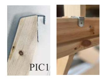
Using the two ladder hooks now attach to the top of each ladder strut, attaching to the slanted inside cut edge, See PIC1 Locate the hooks and attach using the small screw(L). Now hook the ladder over the side rail, this is designed to be tight to prevent movement. You may need to gently tap with a mallet..
