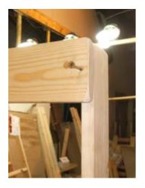
Now Part 11A is in place find the two front guard rails. Red is located at the top, white at the bottom. Now attach to the corner post, level, then again screw in from the inside using the long black screw.
