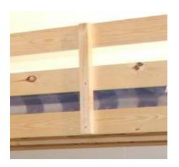
These two rails prevent the guard rails from being forced apart, very important. Using a tape measure find the centre of the back guard rail and centre of the front guard rail. Make a small pencil mark. Then attach each guard rail support to the front using base slat screw (E) provided. These cover both the two guard rails and secure onto the side rail.
